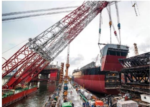
Turret block being lifted into position at front of TEN FPSO, during construction in Jurong shipyard, Singapore
