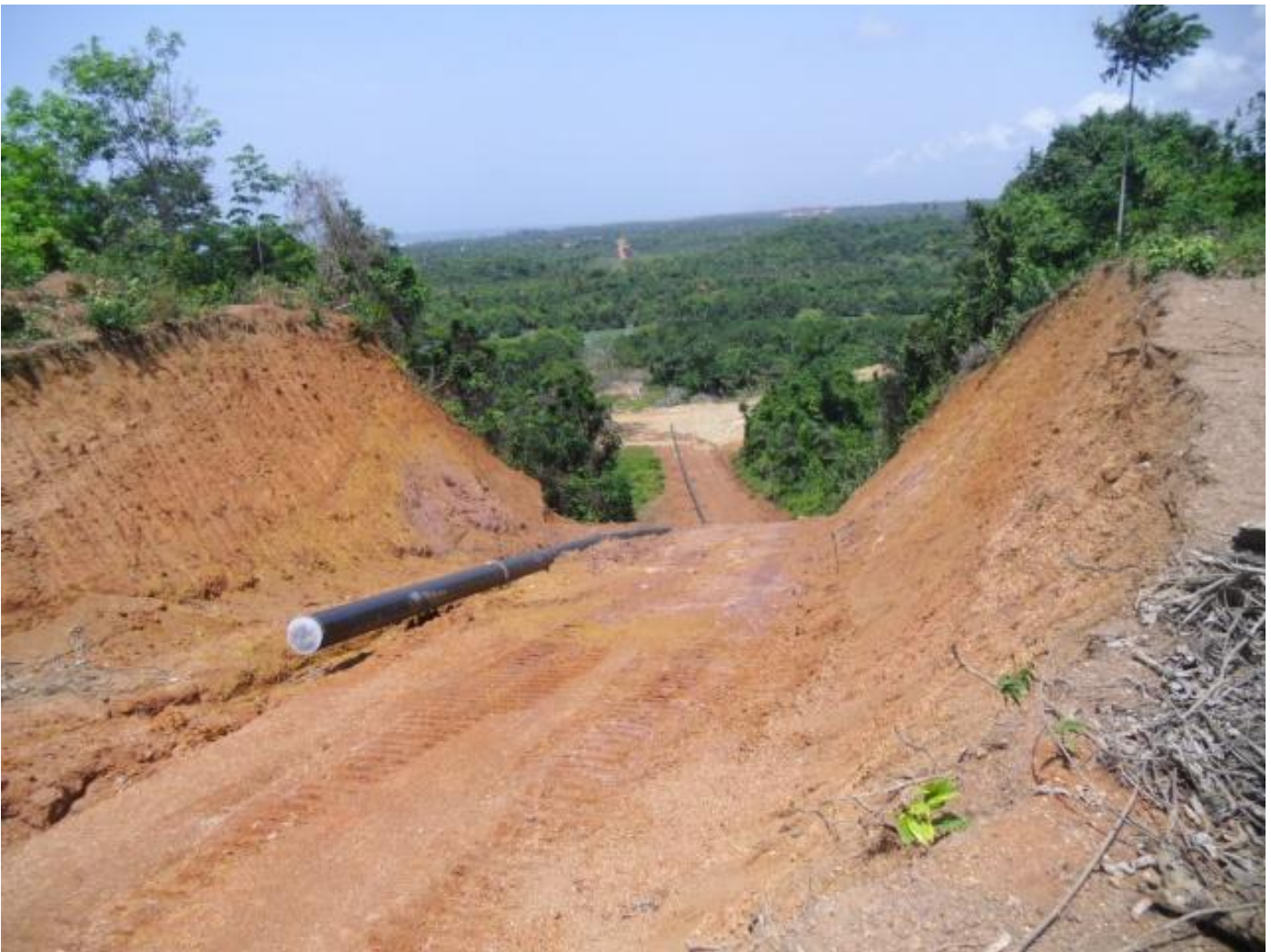
A gas pipeline being laid at the Ghana National Gas project site
